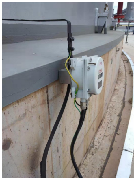
Site installation picture of non-explosion-proof grounding resistance detector
